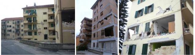
Fig. 1: Examples of in-plane and out-of-plane seismic damage to clay unit masonry infill walls
