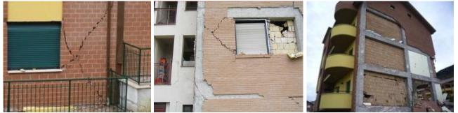
Fig. 2: Examples of in-plane and out-of-plane seismic damage to clay brick masonry veneers
