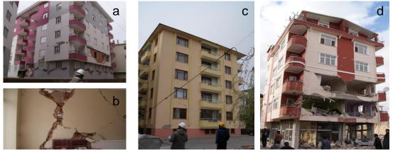
Fig. 4: Damage to infills in 2011 Van Earthquake: a) in-plane damage, b) damage inside building in a, c) moderate damage, d) heavy combined damage
