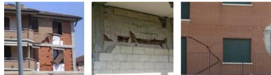
Fig. 5: Masonry infill and veneer damage: Emilia, Italy, 2012
